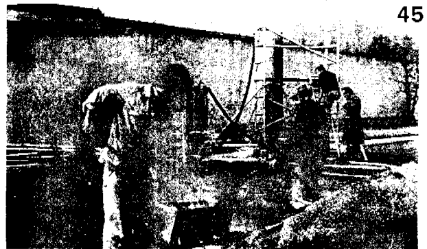
Cyclone for gravel washing. Trial operation in the Lakewater Plant Moos.
