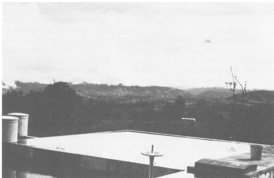
SSF Filter in Alto de los Idolos, Colombia at the beginning of flow testing.
