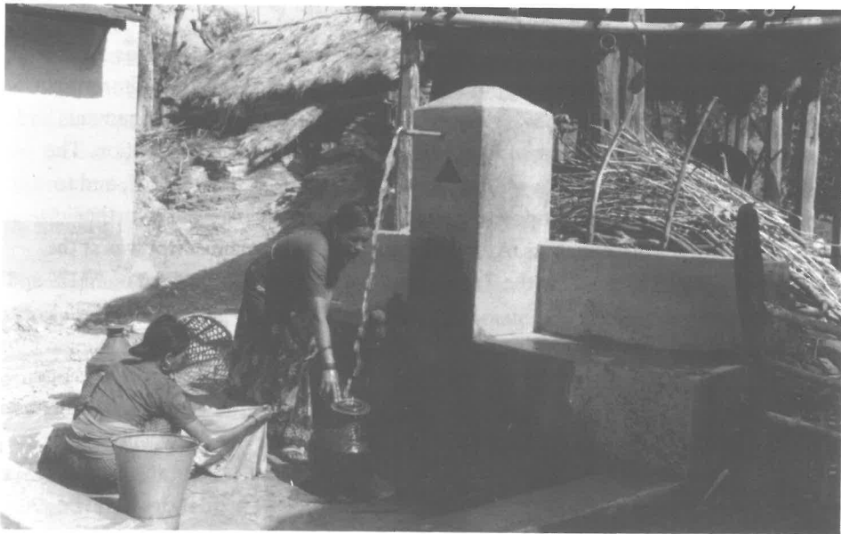
A newly constructed tapstand in the Western Development Region in Nepal being used for washing and drinking water collection. (photo IRC)
