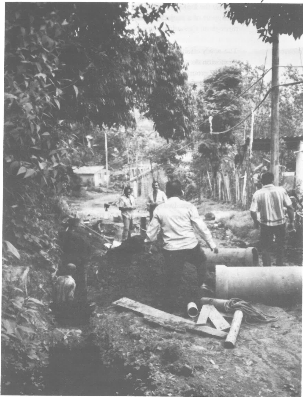
Community involvement in sewerage construction in Colombia.
