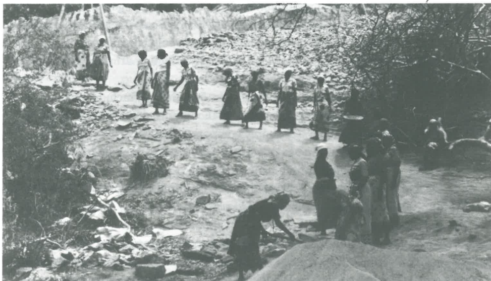
Womens Mwetthya self-help group participates in the construction of a village rock catchment dam at Mitono, in Kitui district, Kenya.
