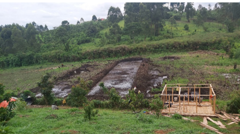
Supervising and monitoring of the construction of standard earthen ponds in Kiko TC.
