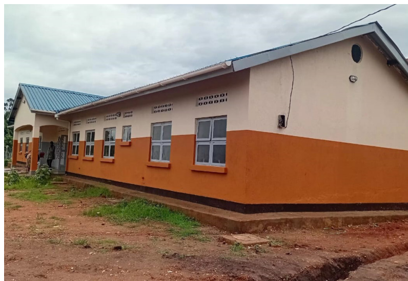
The newly constructed general ward at Kituule HCIII in Hakibale Sub county
