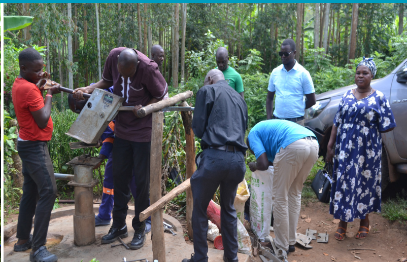
A section of district works committee of council witnessing borehole repair works in Kicwamba Sub county
