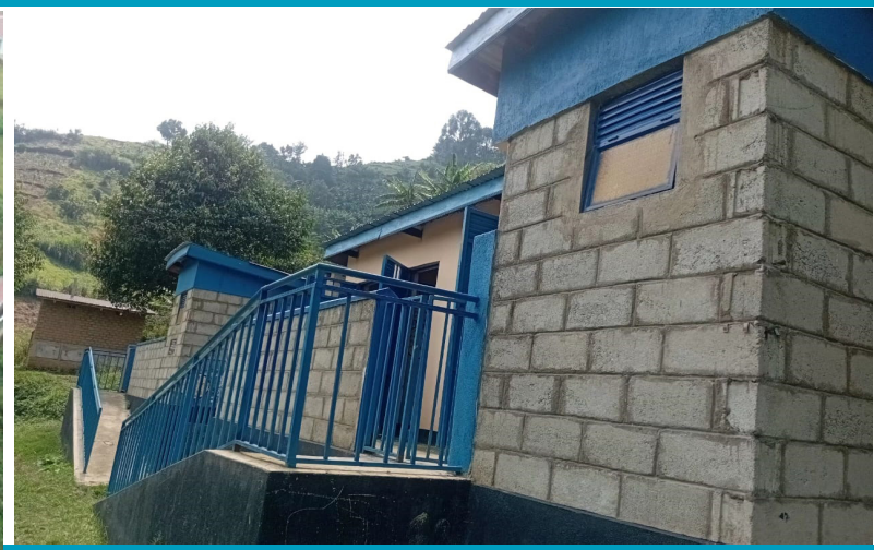
A VIP latrine facility constructed at Mount Gessi Primary School in Karangura Sub County
