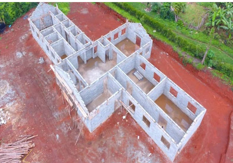
Ongoing construction works for a general ward at Nsorro HCIII in Kijura Town council
