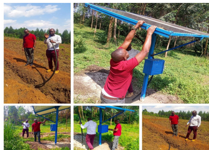
Inspection of Ugift Micro Scale irrigation work by the water Engineer and the Senior Agriculture Officer Kabarole
