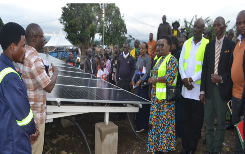
District leaders commissioning the Nyakitokoli solar power plant in Nyakitokoli Parish, Karangura Sub county
