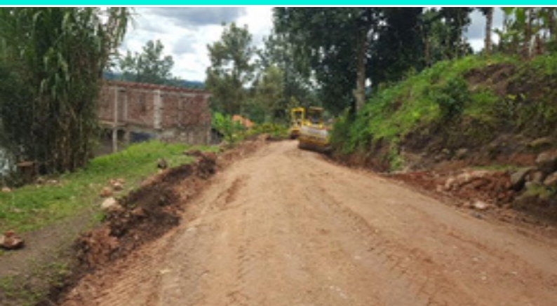
Road works on Rwengaju Katoma Kijura road under Local Economic Growth Support
