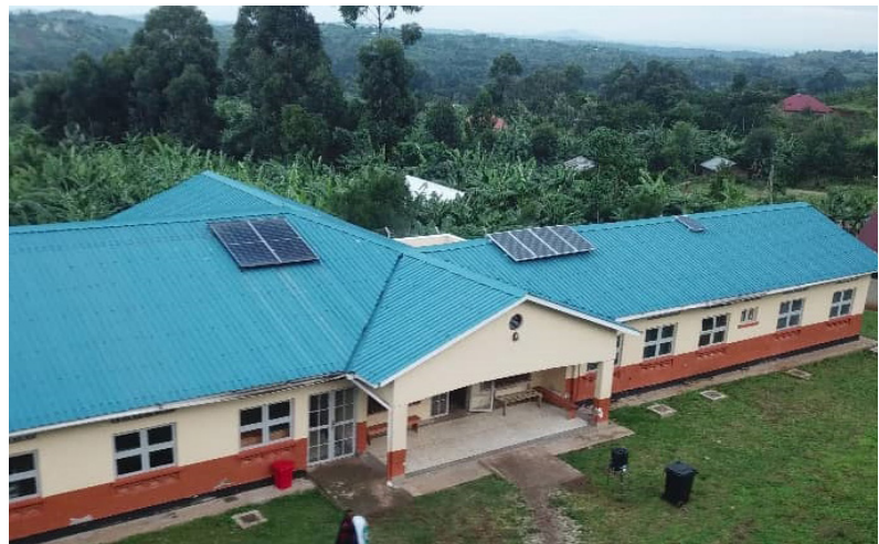
A general ward at Nyabuswa HCIII in Mugusu Sub County
