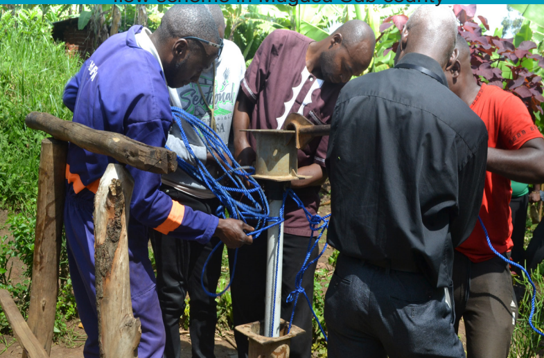
Water Engineers demonstrating borehole repair works in Kicwamba Sub county
