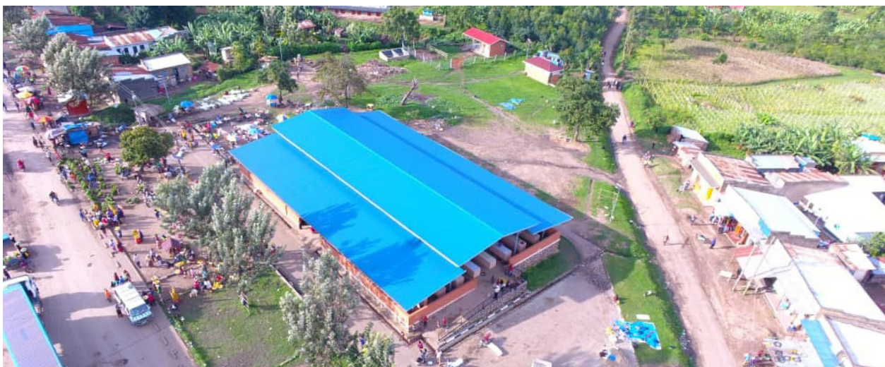
Aerial View of Kihondo Roadside Market constructed under LEGS Project in Kicwamba Sub County
