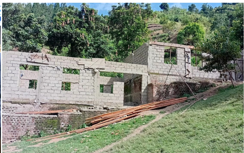
Construction works of a two-classroom block at Mount Gessi Primary School in Karangura Sub County
