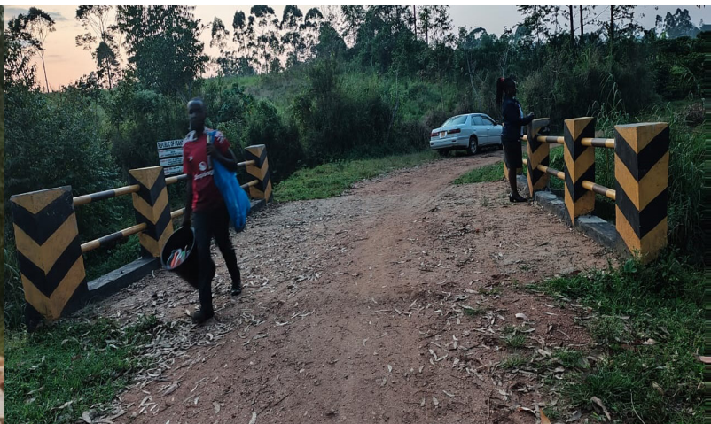
Kisakyabairu bridge after construction in Busoro Sub County
