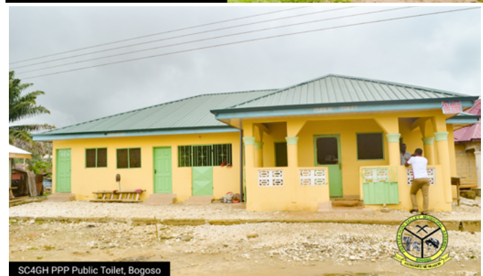
SC4GH PPP Public Toilet, Bogoso
