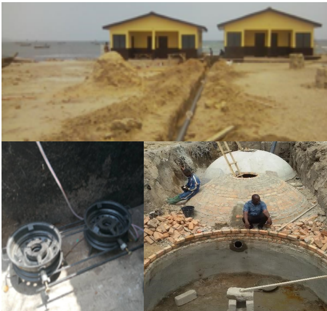
Gas line back to prisons (top), gas used at prisons kitchen (bottom left) and construction of biogas toilets (bottom right)..
