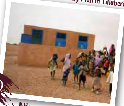
Toilet block well built by Plan in Tillaberi
