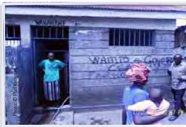
Toilet constructed in Motherland, Kamukunji , Nairobi .
