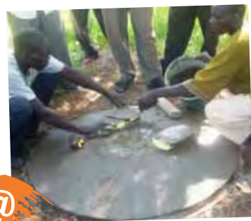
Construction of low cost latrines in Tororo, Uganda
