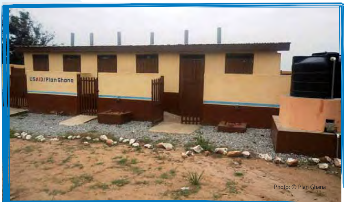
New toilet facilities at Mpota Junior High School in Ghana
