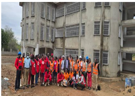
Figure 2-10: Team inspection of the office block under construction
