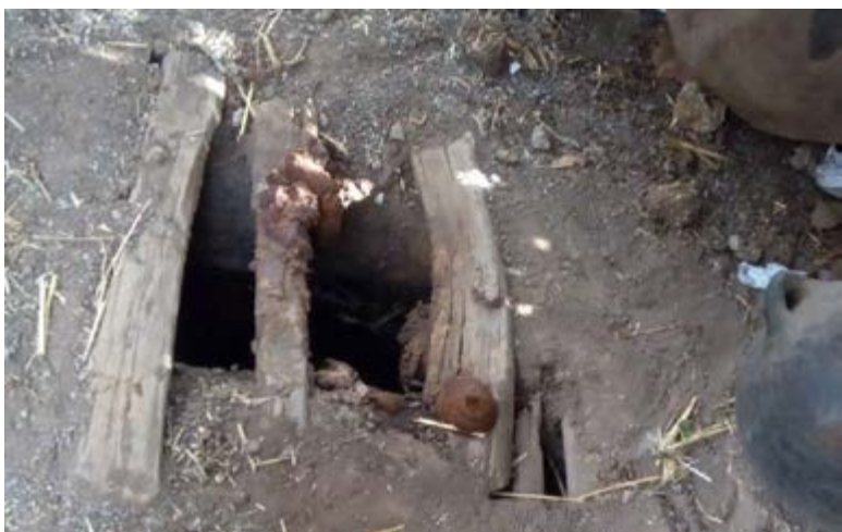
Figure 4 – Unimproved pit latrine
