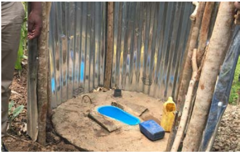
Figure 5 – Improved pit latrine
